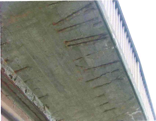
BETONABPL RE
